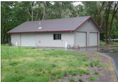
Large shop with 3 rollup doors.
